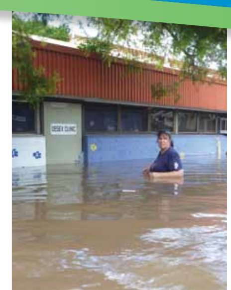
Floodwaters inundated three-quarters of the Fairfield Shelter.
